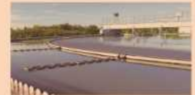
Improved Sewage Treatment
